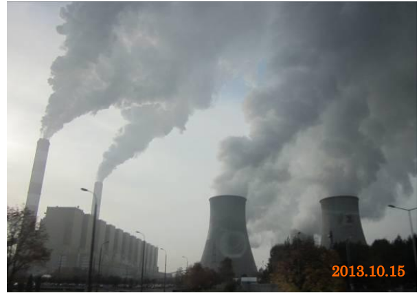
Belchatow Power Station
