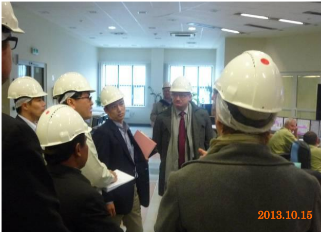
Checking the operation status in the main control room (Belchatow Power Station)
