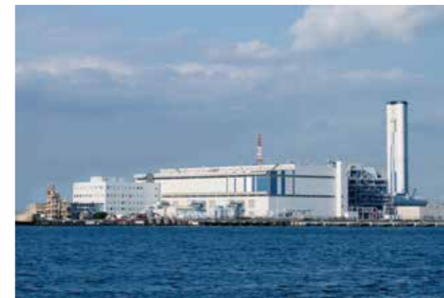
Kawasaki Thermal Power Station (LNG Combined-cycle)
