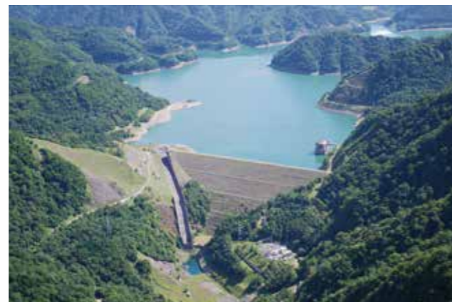
Takami Hydroelectric Power Station
