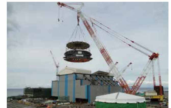
Ohma Nuclear Power Station (ABWR, Under Construction)
