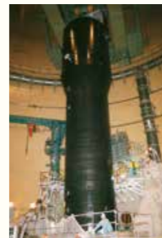
Steam generator of Mihama Unit 3 being replaced
