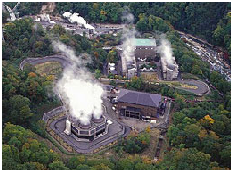
Kakkonda geothermal power plants Tohoku Electric Power Company Co., Inc., Japan
