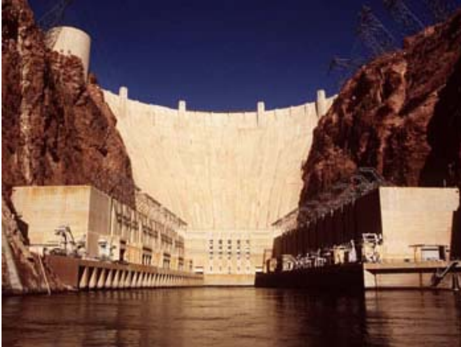
Conventional Hydropower – Hoover Dam
