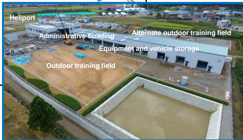
Construction status of the new base (As of November 4, 2016)
