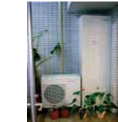
EcoCute Heat Pump Unit (left) and Hot Water Storage Tank
