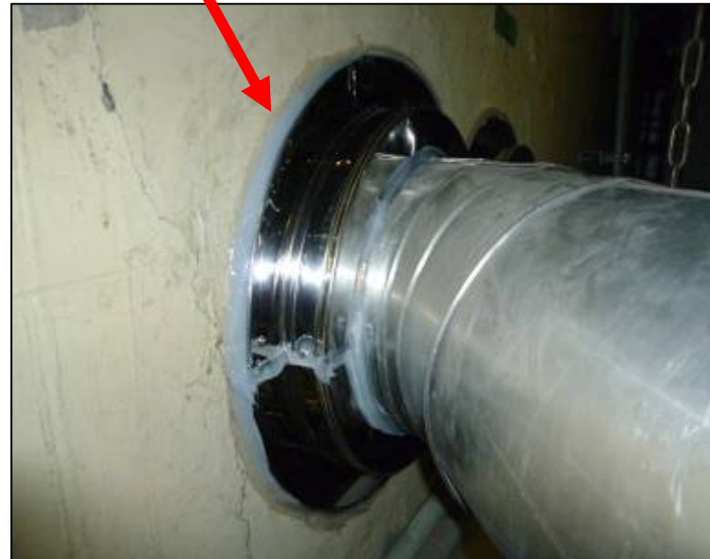
Sealing for pipe penetration part
