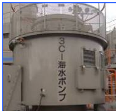
【Deployment of a backup seawater pump motor】 (scheduled to be deployed in March 2012)
