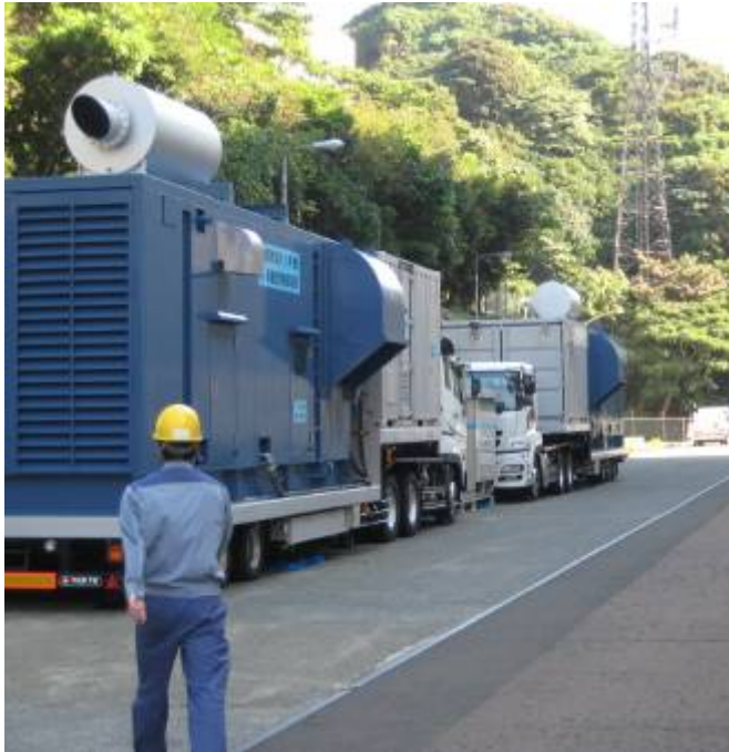
Emergency air-cooled generators
