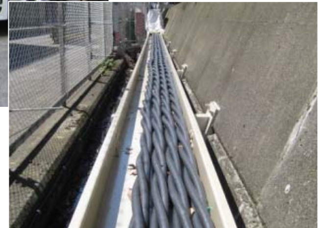
Installation of cables
