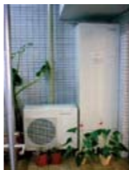
EcoCute Heat Pump Unit (left) and Hot Water Storage Tank
