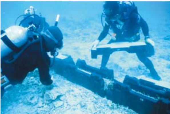
Laying Operation of Submarine Cable
