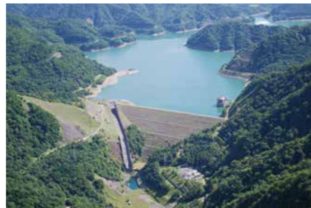
Takami Hydroelectric Power Station
