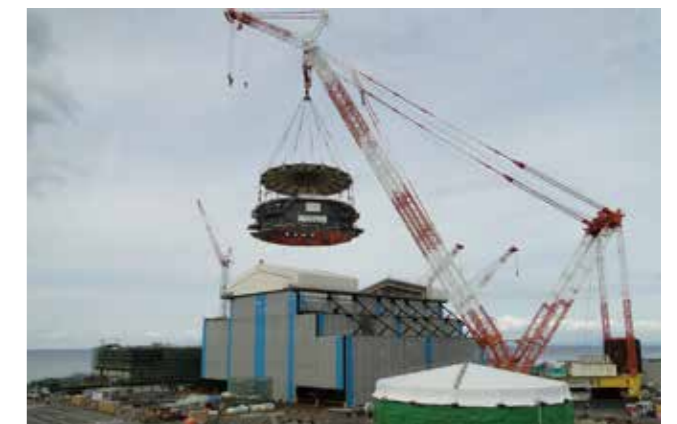
Ohma Nuclear Power Station (ABWR, Under Construction)
