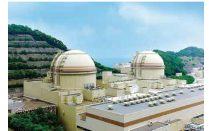
Ohi Nuclear Power Station (PWR)
