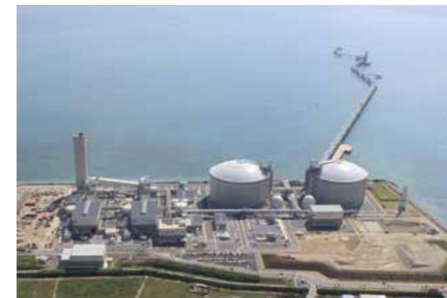
Yoshinoura Thermal Power Station (LNG-fired)
