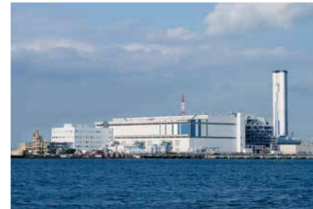
Kawasaki Thermal Power Station (LNG Combined-cycle)
