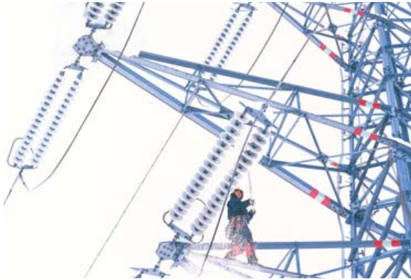
Snow removal for transmission lines
