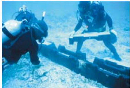
Laying operation of submarine cable
