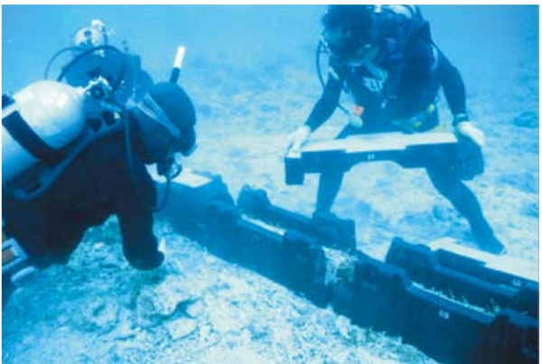
Laying operation of submarine cable
