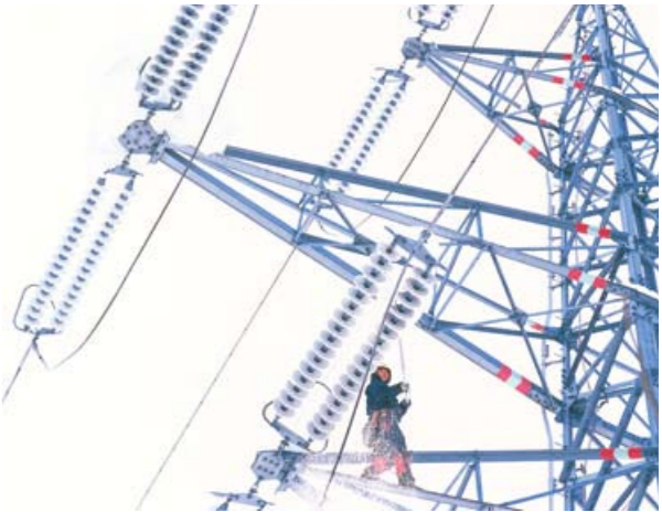
Snow removal for transmission lines
