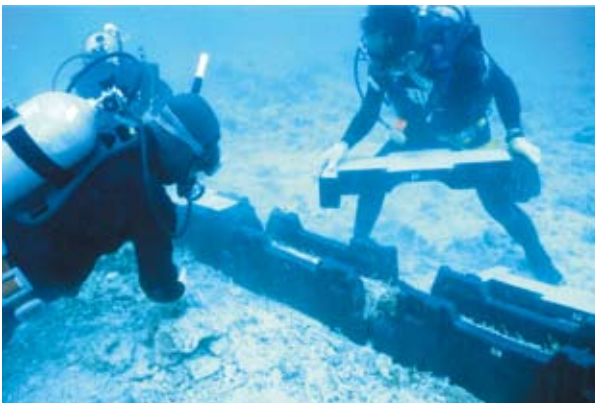
Laying Operation of Submarine Cable
