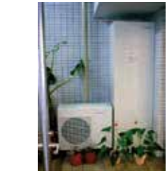
EcoCute Heat Pump Unit (left) and Hot Water Storage Tank
