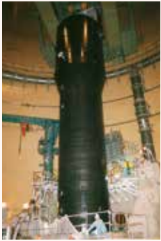
Steam generator of Mihama Unit 3 being replaced
