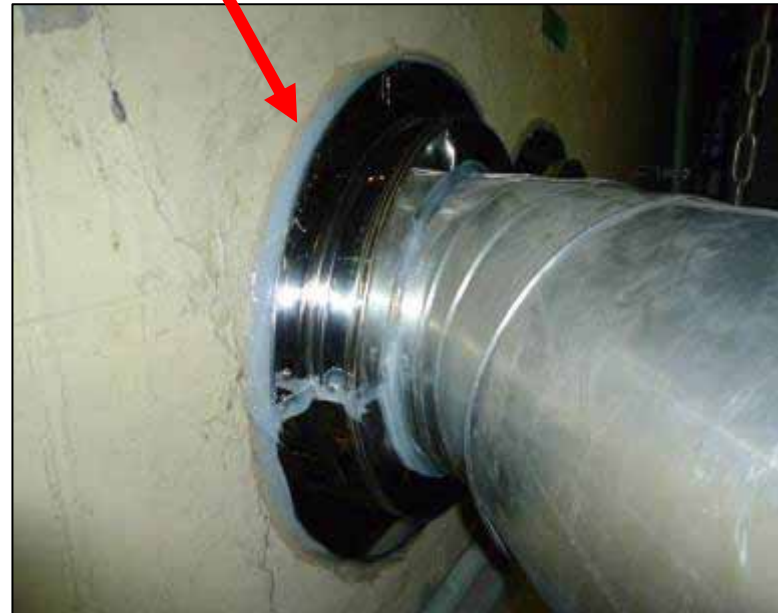
Sealing for pipe penetration part
