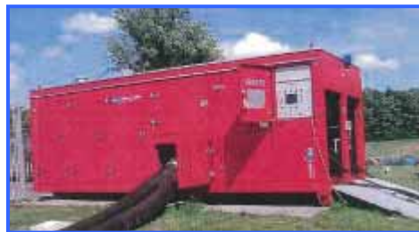
【Deployment of a large-capacity temporary seawater pumps】 (scheduled to be deployed in December 2011)
