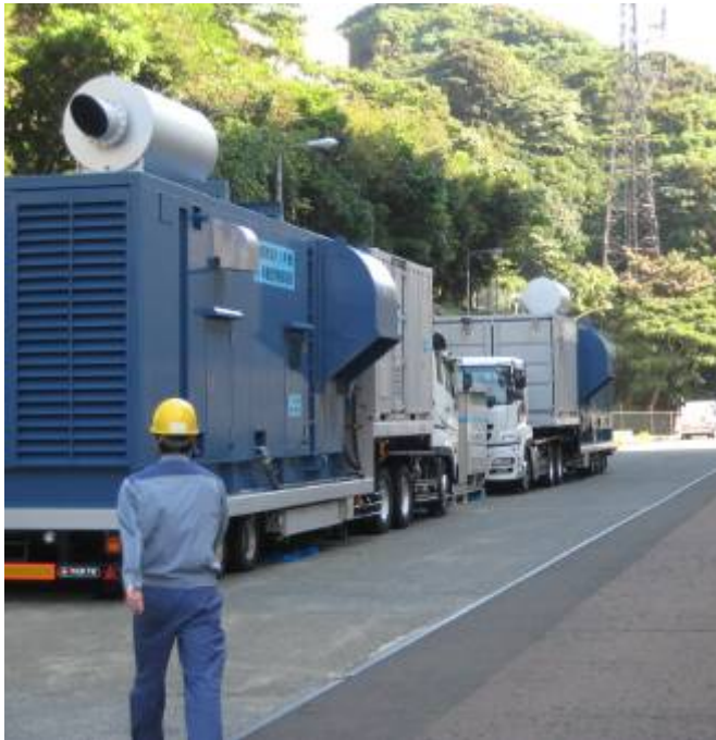
Emergency air-cooled generators
