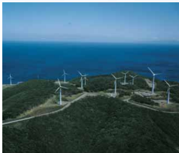
Tappi Wind Park, Tohoku Electric Power Co.
